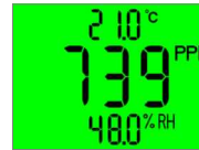
Diagram 3 When switch 2 is in the downward position with the Temp & RH Module attached then the Temp & RH will be displayed.
